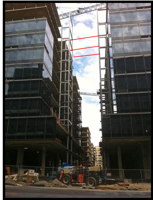
Figure 15: Structural Steel Frame for Bridges
